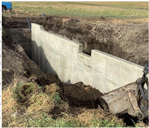
CD 61 storage and treatment wetland weir structure shortly after the forms have been removed.
