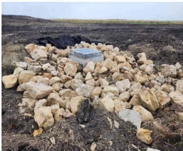
Water control structure and rip rap
