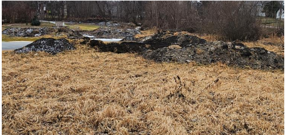
A WCA violation site where a landowner left spoil piles in the wetland.
