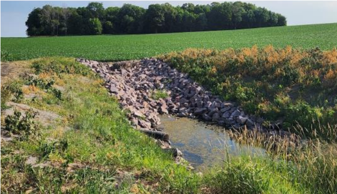
Grade Stabilization Structure
