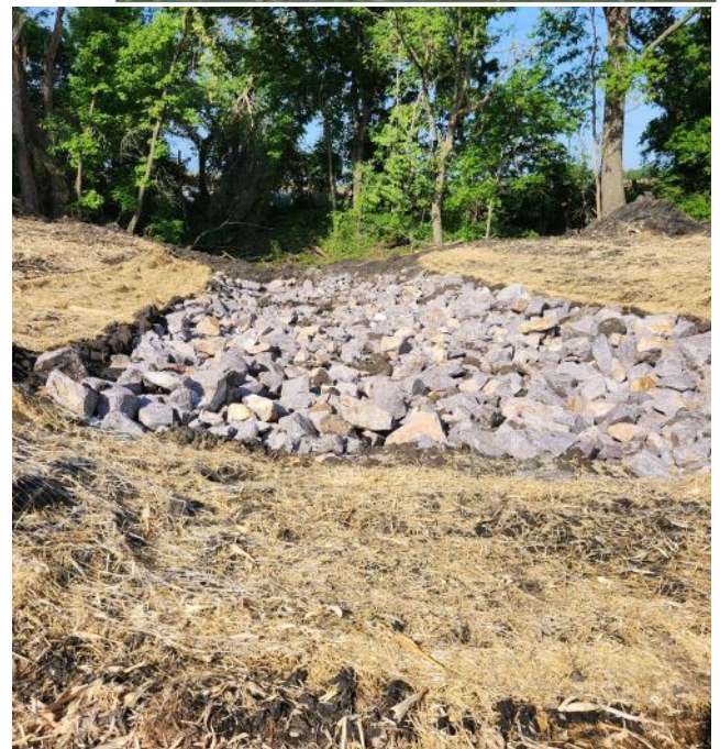
Grade Stabilization Structure Construction –Spring 2023
