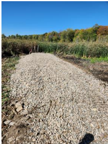
Rock Access Road
