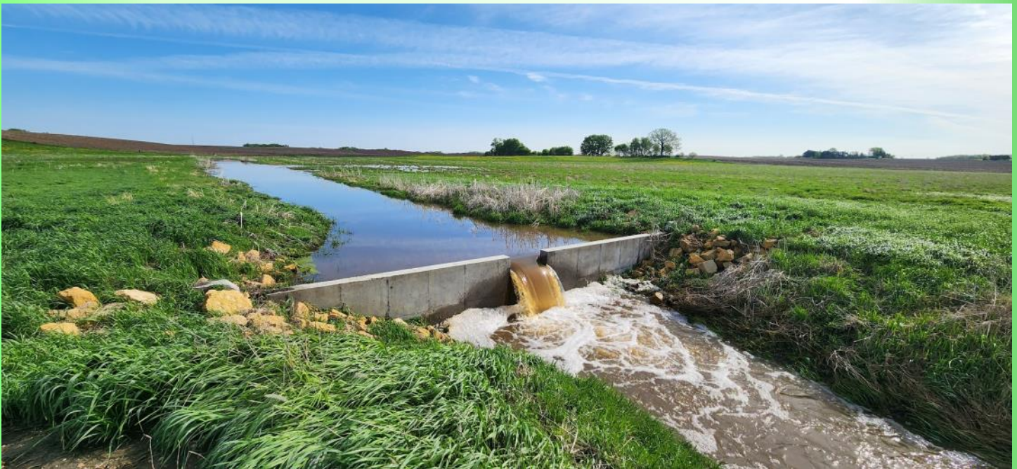
Multi-Purpose Drainage Management Water Storage Outlet after a 5" Rain Event Spring 2023
