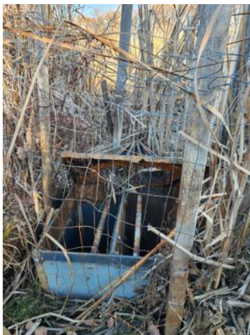
Existing Agri Drain Structure
