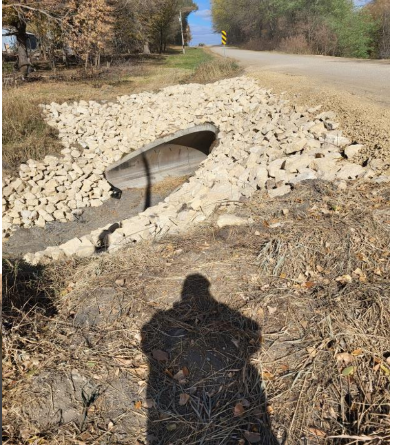
CD37 Culvert repair and armor project in Cleveland Township.
