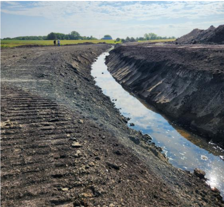
Surface ditch reroute completed
