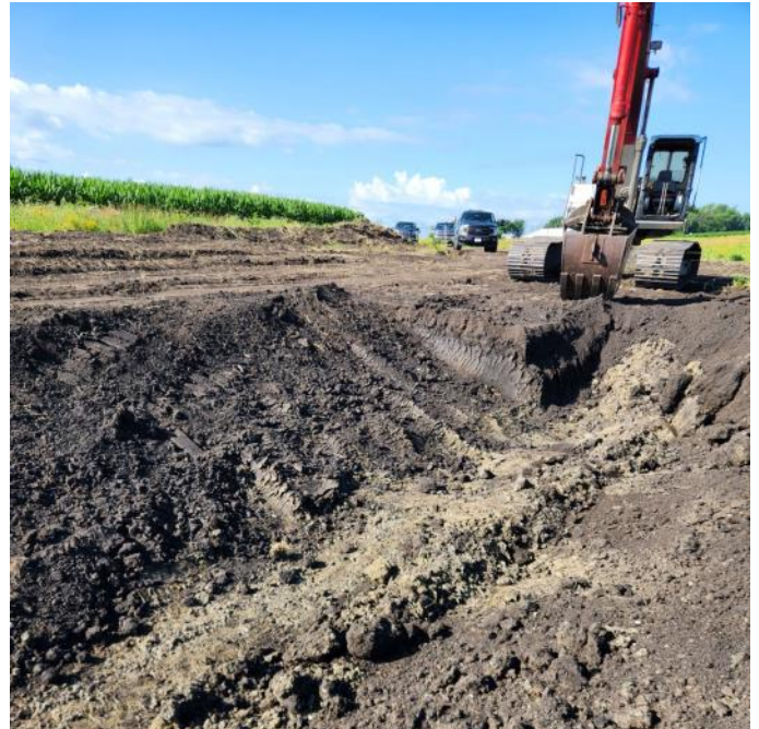
Digging surface ditch reroute
