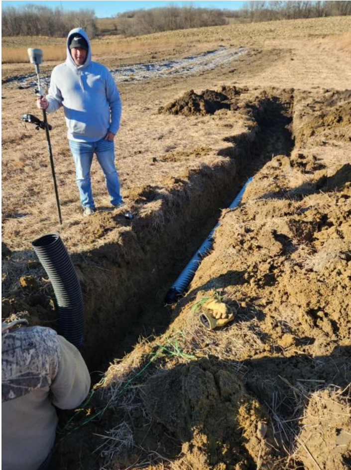
Tile Break & Reroute
