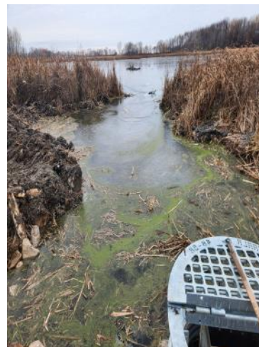
Excavated Channel to Structure
