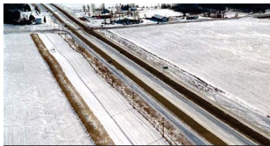
A Living Snow Fence in use along a major four lane highway in Minnesota
