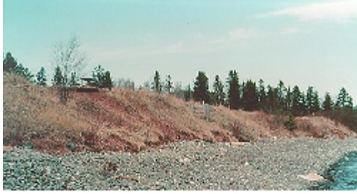
The shoreline at this Two Harbors campground was severely eroded...
